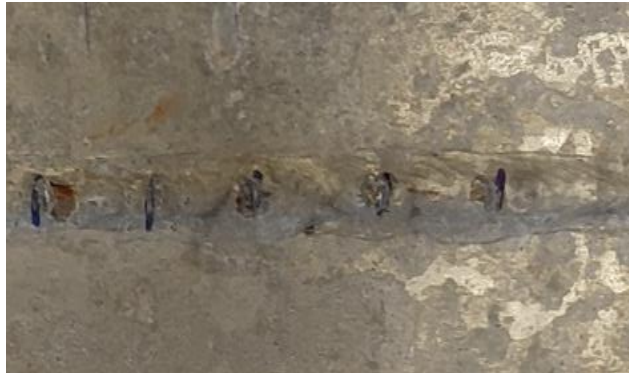
Figure 8 Photograph of the sample after the condensation chamber test.
