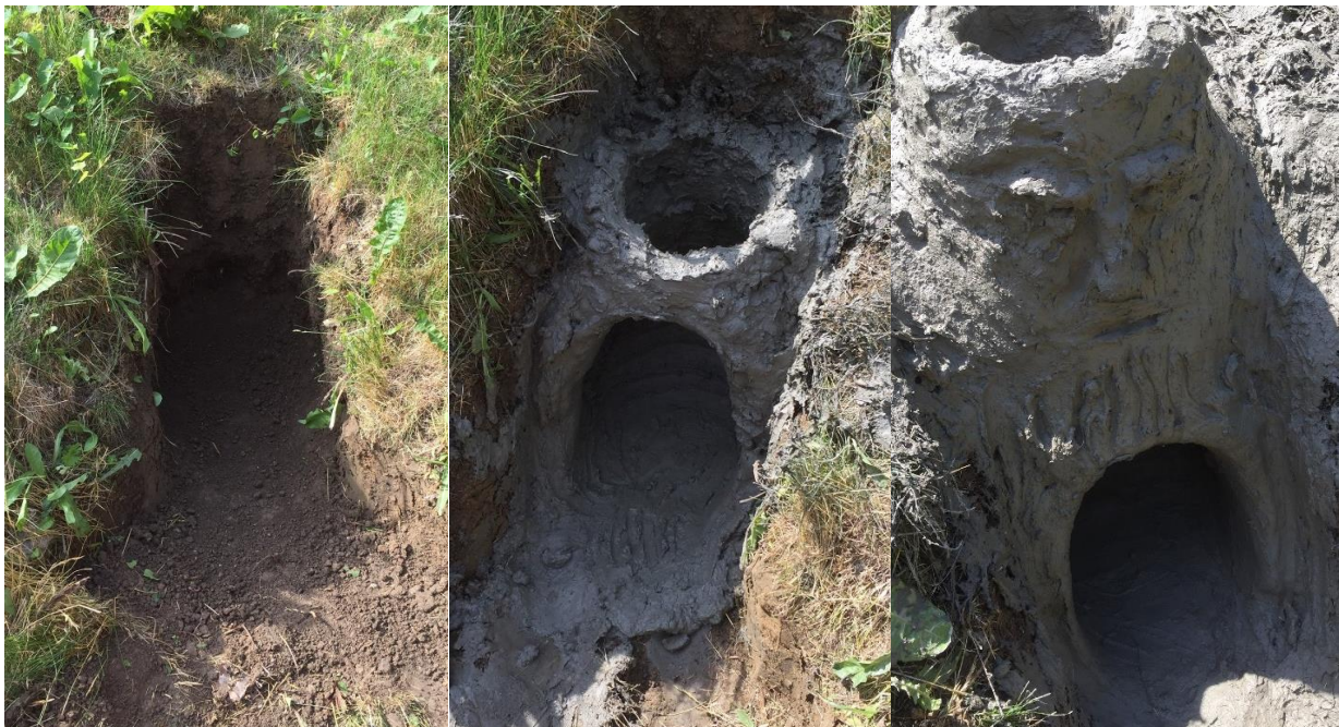
Figure 3 From left to right: a – Dug out groove, b – the arc of the entrance, c – finished furnace.
